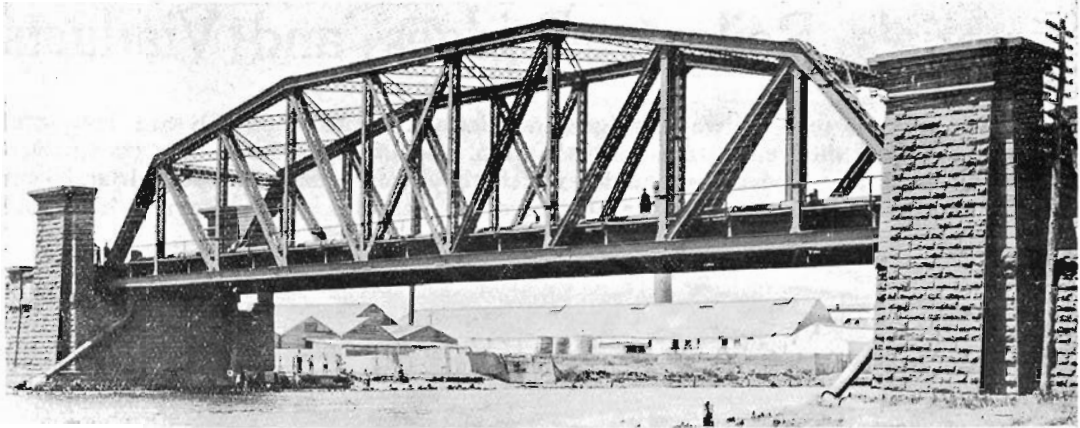
This Bridge, which spans the Saltwater River, mid-distance between South Kensington and Footscray, is a fine example of engineering skill.
