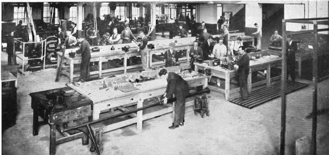
View of portion of the new workshop recently taken over by the Electrical Superintendent.
