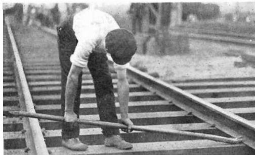
Correct method of holding claw bar when pulling out dog spikes.
