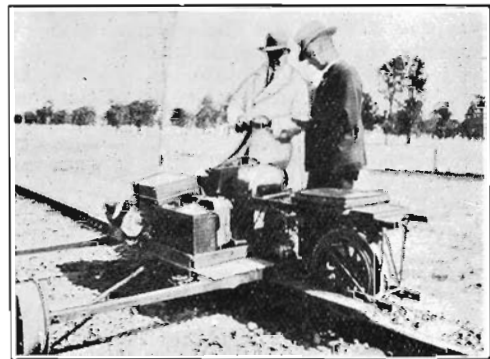
The Joys of Motoring—Messrs. Abraham, Traffic Inspector, and Nolan, Roadmaster, (white coat), repair a broken belt between Murtoa and Jung.
