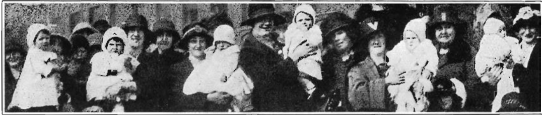
Splendid work is being done by the Baby Health Centres Association Staff on the Better Farming Train. Here's a fine group of babies taken when the train visited Bungaree.
