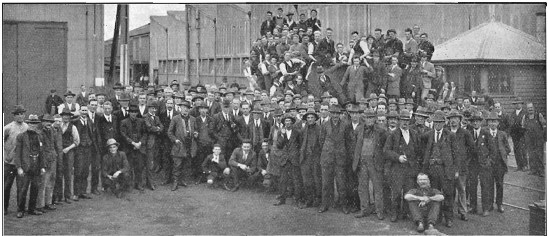
Some of the 400 odd men who are employed at the well-equipped Signal Shops, Newport, where all sorts of signalling and interlocking apparatus, and railway telephone, telegraph, and safeworking devices are manufactured.
