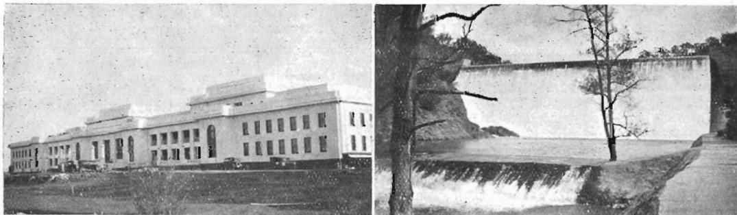
On the left is the new Parliament House at Canberra, the new Federal Capital, where the Duke and Duchess of York will open the Federal Parliament in May next year. On the right is the Cotter Weir. By damming the Cotter River sufficient water has been impounded to supply the needs of the new Federal City for sixty or seventy years. Provision has been made to increase the area impounded as the population increases.
