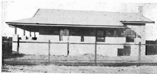
One of the fine departmental residences being erected for railwaymen at Balranald.
