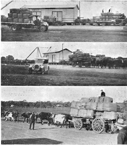
Three "snaps" taken in Balranald railway yard, showing the modes of transport utilised there.
