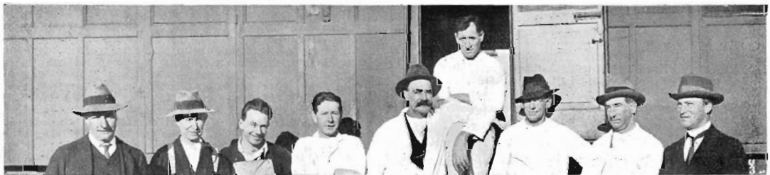
Some of the painters and carpenters who have just completed the seven weeks' job of renovating the Warragul railway station. On the extreme right of the group is Mr. R. J. Withey, Acting Works Foreman.
