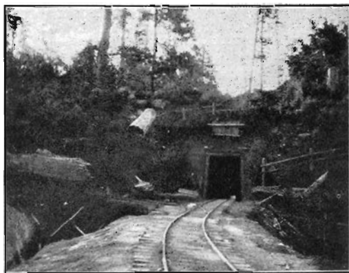
Few people know that there is a narrow-gauge railway operating in the hills not 70 miles from Melbourne, and that a tunnel 1000ft. long has been cut through the Dividing Range to enable the timber to be conveyed to Powelltown. The line was constructed and is owned by the Victorian Timber Company.
