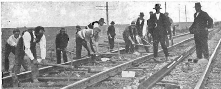
Some of the gang at work relaying the track between Melbourne and Seymour.
