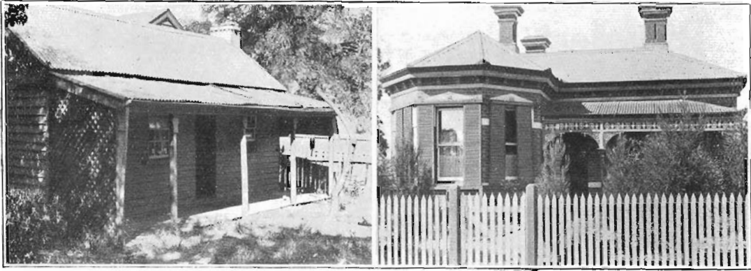
Conclusive proof of Seymour's progress is afforded by a comparison of these two photographs. The one on the left is the first stationmaster's residence, built in 1870, and the other is the fine home of the present S.M. (Mr. J. C. Boyd). The old residence is about to be pulled down to make way for the new Institute Rooms.
